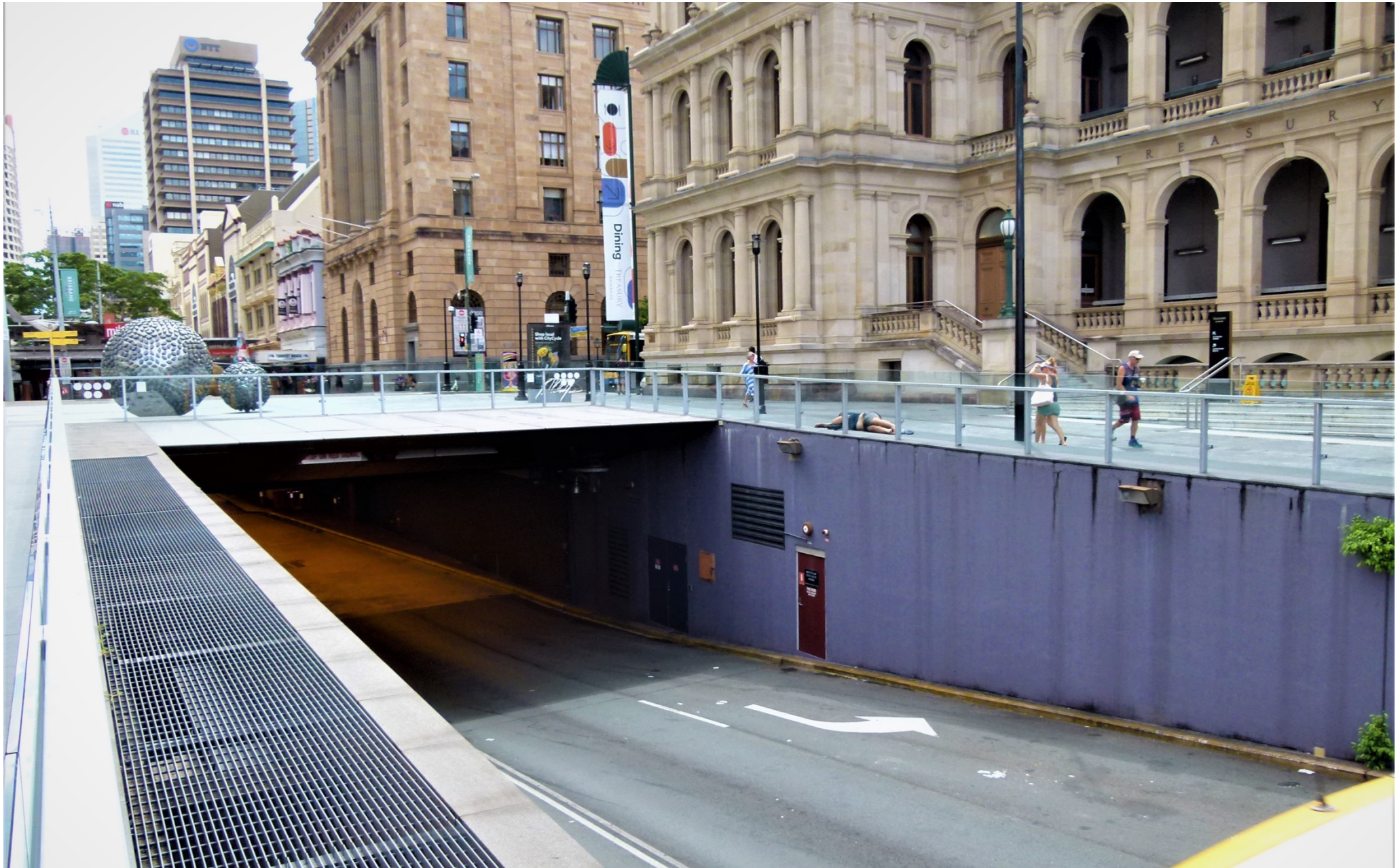
Fig.3b Portal to Queen St busway station access tunnel
