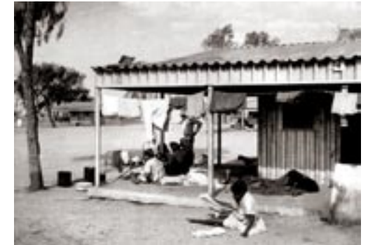
Aluminium shelters at Amoonguna near Alice Springs
