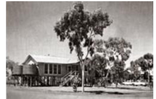
Below: Staff house at Warrabri settlement, Northern Territory
