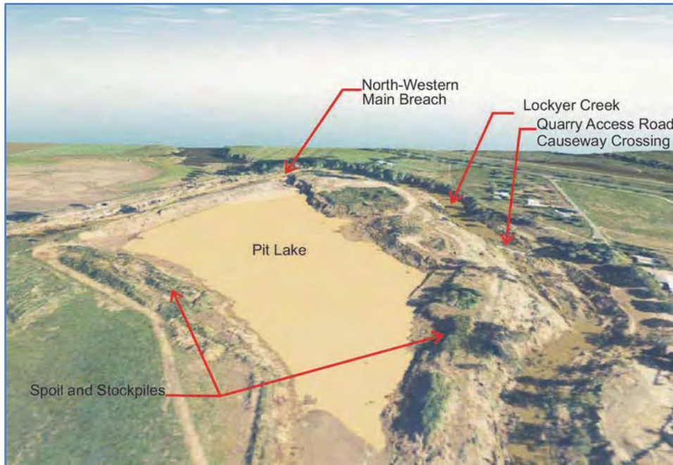
Figure 5.11: Oblique view after 10 January 2011
